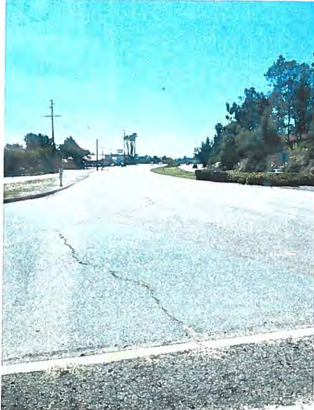
Figure 4. North intersection - looking south
