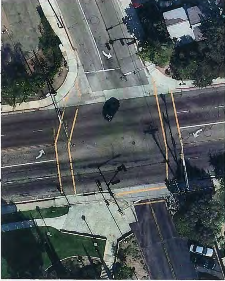
Escondido High School Sidewalk Expansion (before)
