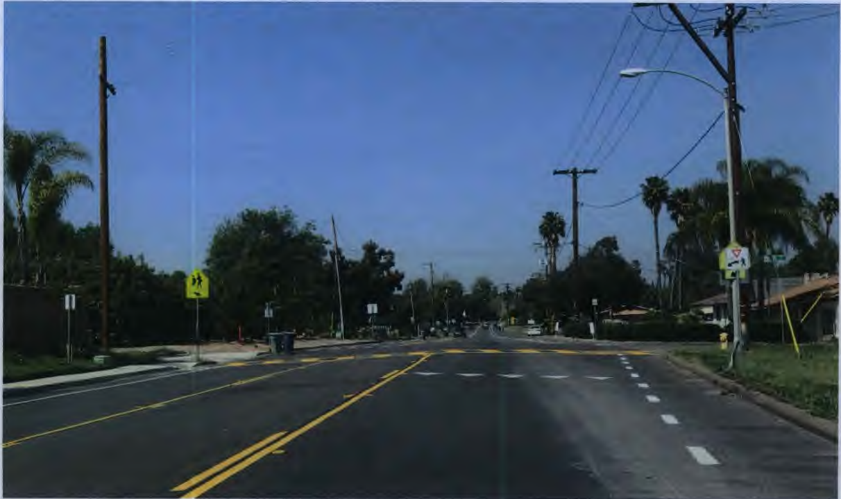
Figure 4 – New Striping Installed on Felicita Road
