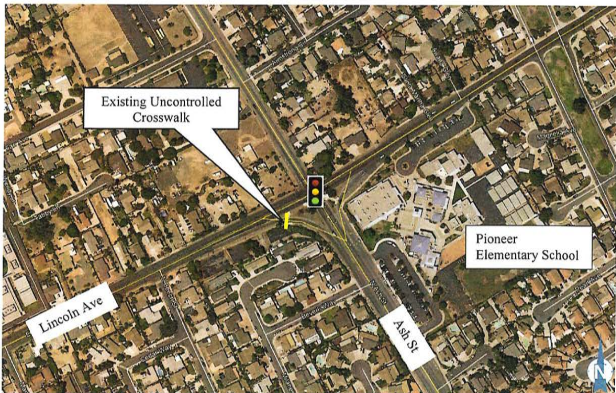
Figure 5 - Uncontrolled Crosswalk at Lincoln Avenue and Ash Street
