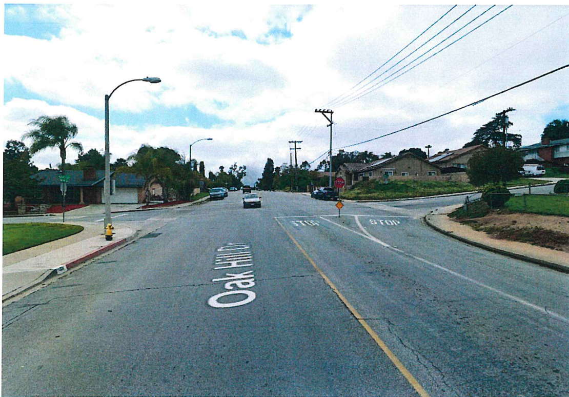
Figure 6 – Existing Condition of Rose Street and Oak Hill Drive Intersection
