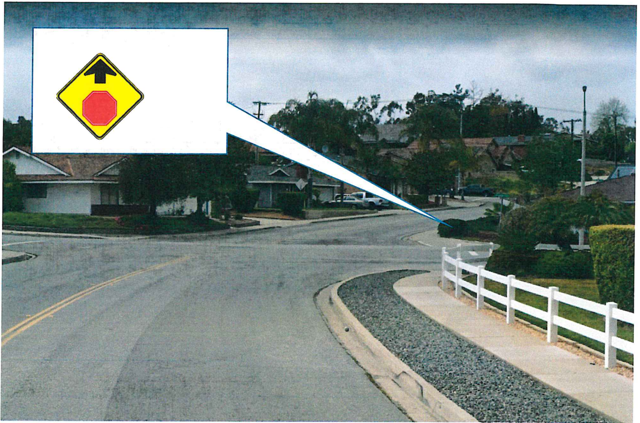
Figure 6: Existing Stop-sign may be difficult to see due to horizontal curve. New Stop-ahead signage will alert northbound drivers.
