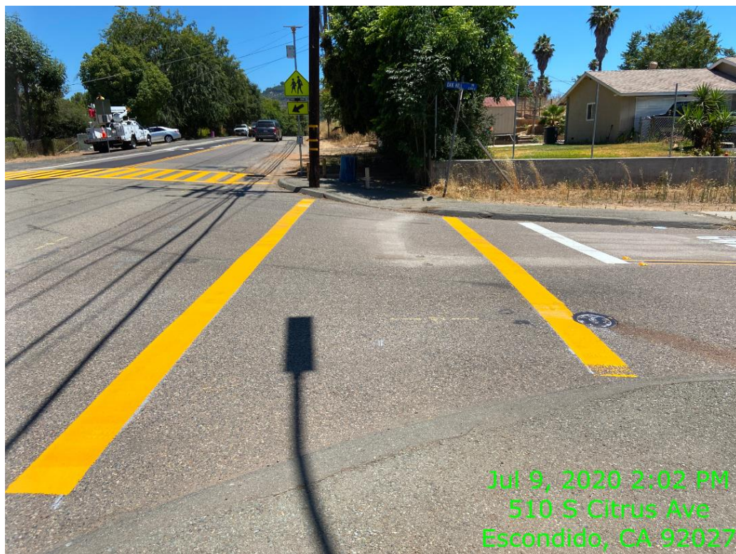
Figure 6: Crosswalk on Oak Hill was also refreshed.
