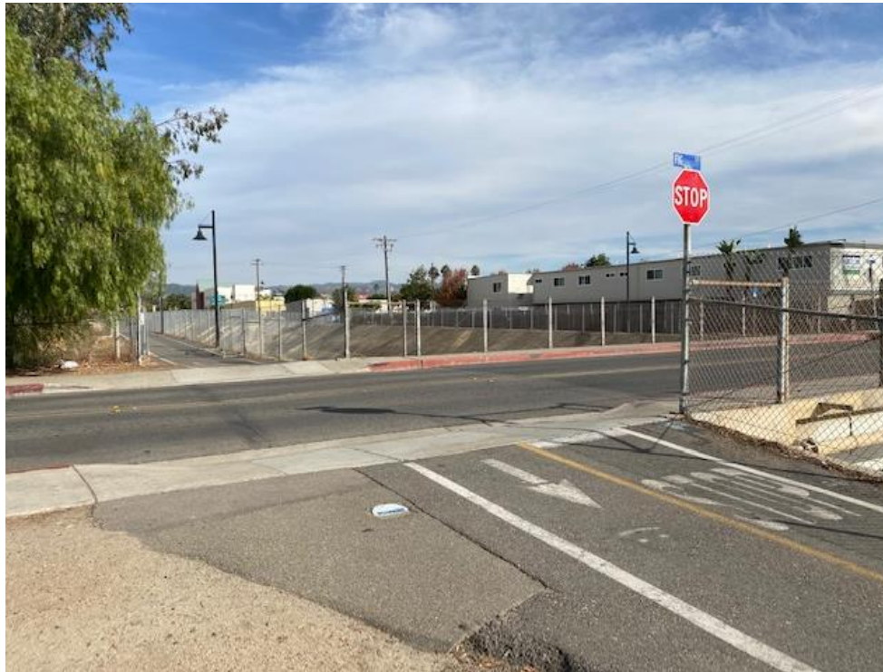
Figure 6: Existing conditions at Fig Street.
