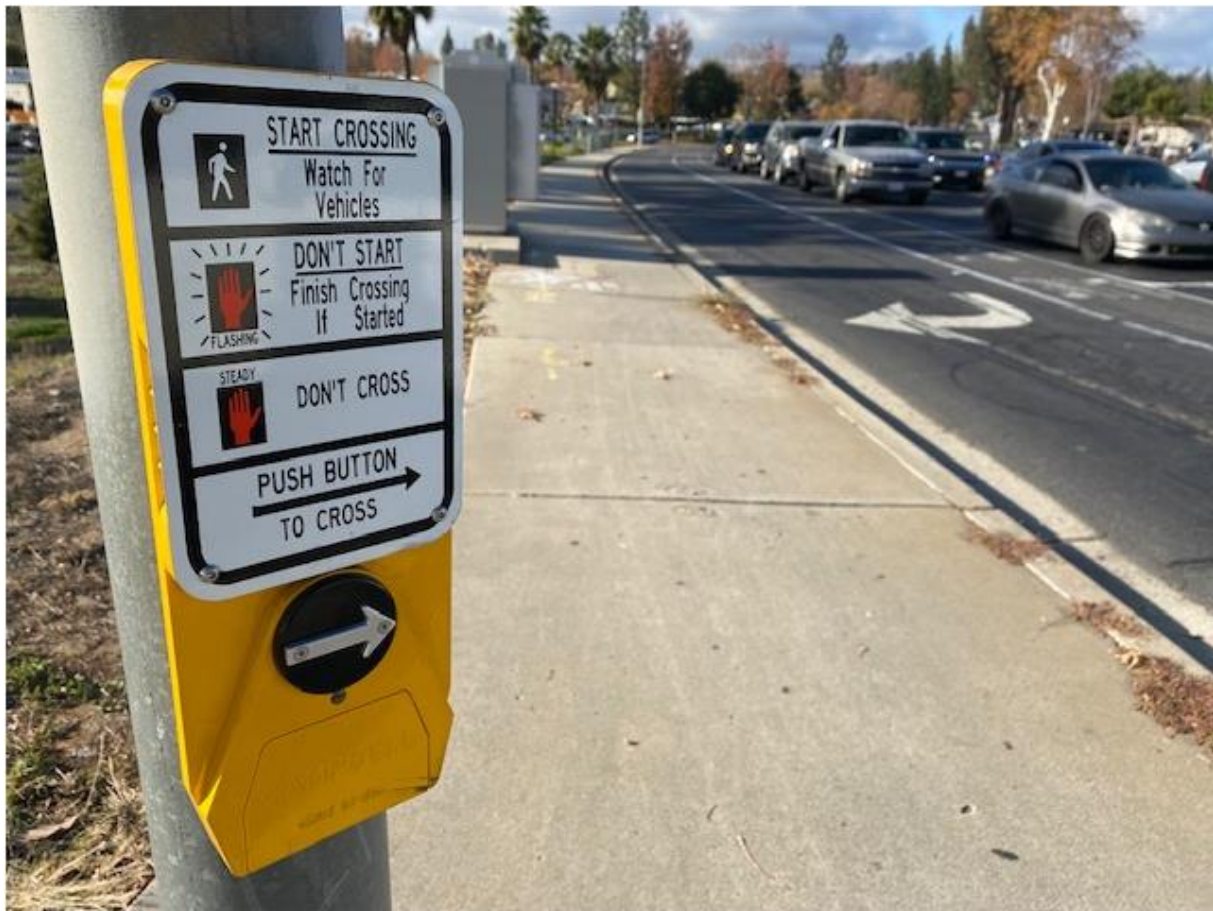
Figure 17: At El Norte Parkway, pedestrian push-buttons were replaced with 8 new APS units using TMPL-funding.
