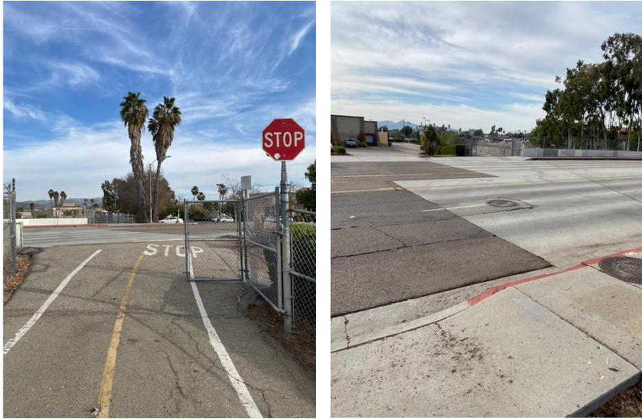
Figure 8: Existing conditions at Harding Street.
