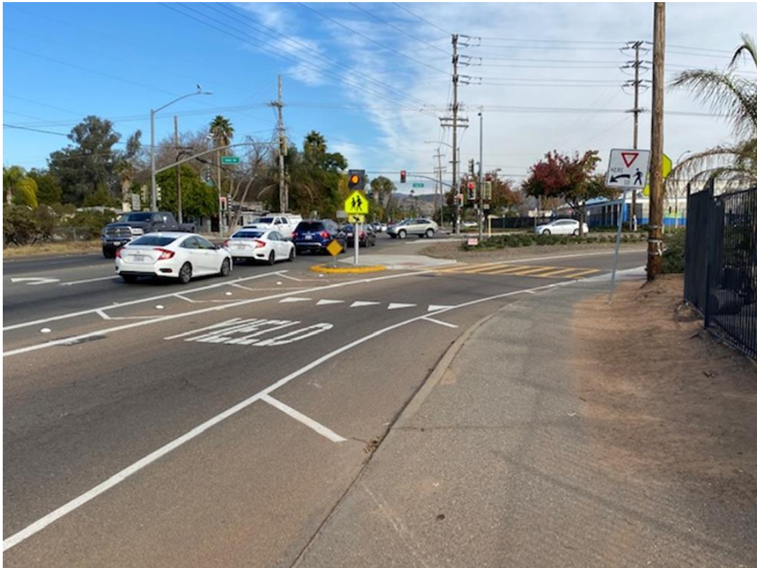
Figure 12: Palm tree was removed, new striping, signage and bollards are in place.
