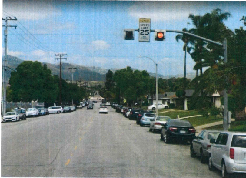
Figure 9: Flashing beacons are installed for both approaches to inform drivers of school speed limit during arrival and dismissal times. Additional beacons are not proposed.
