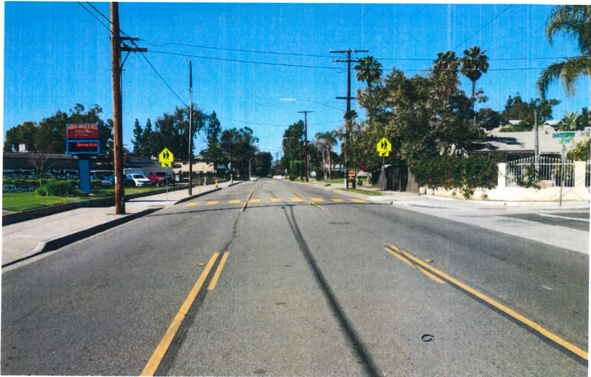
Figure 2: Current conditions at Mission Middle School's Mid-Block Crosswalk.
