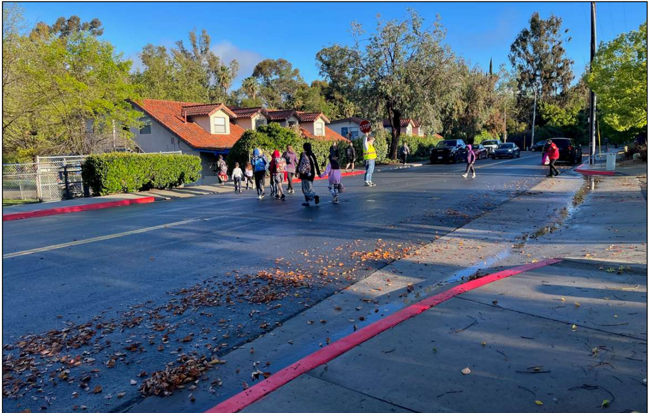
Figure 34: Red curb was added to improve pedestrian visibility in the crossing at Canyon Road and Gretna Green Way
