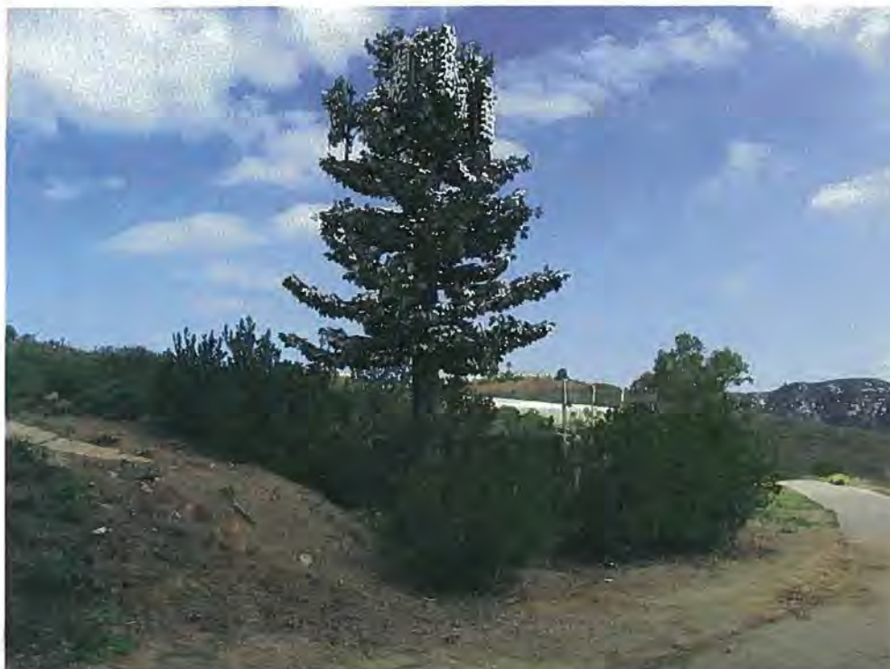
Figure 3: T-Mobile Antennas #13 through #18
