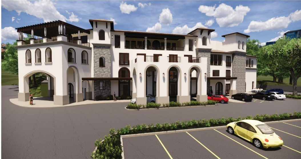
1 ASSISTED LIVING ENTRY FROM PARKING LOT
