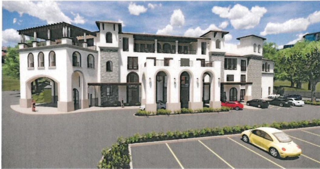
1 ASSISTED LIVING ENTRY FROM PARKING LOT
