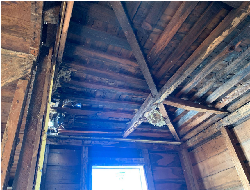
Figure 6. Note “Blackened” appearance on framing, this is evidence of extreme dry rot. Also note the limited framing support members and improper connection, all which increase likelihood of collapse.
