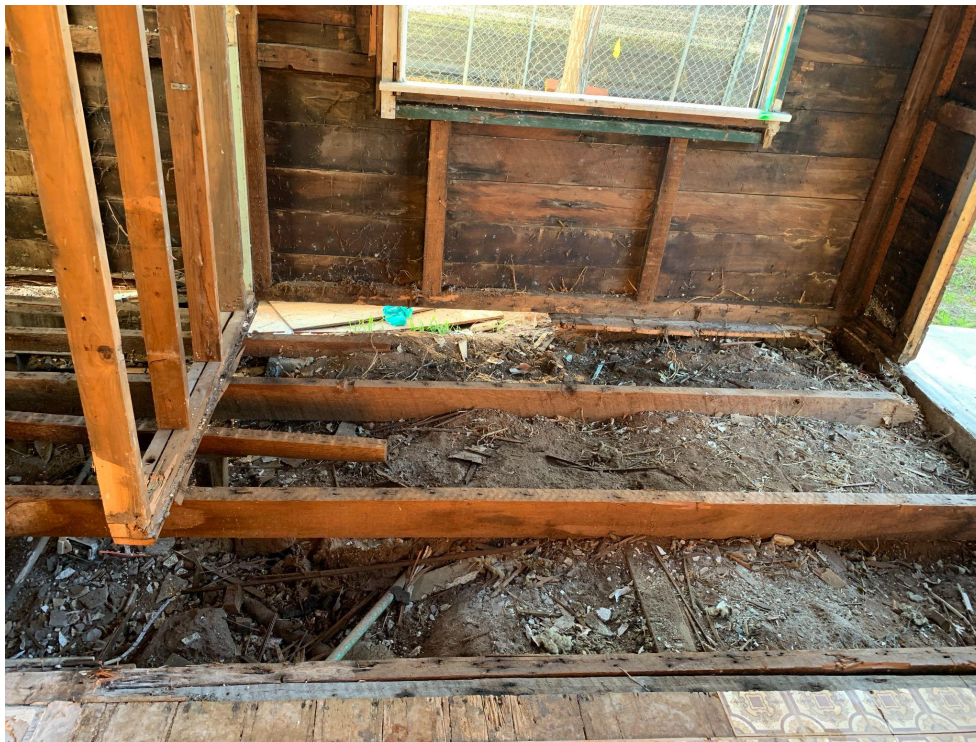
Figure 4. Interior View ( no support below exterior wall. Floor joists are unsupported and sitting directly on soil.)
