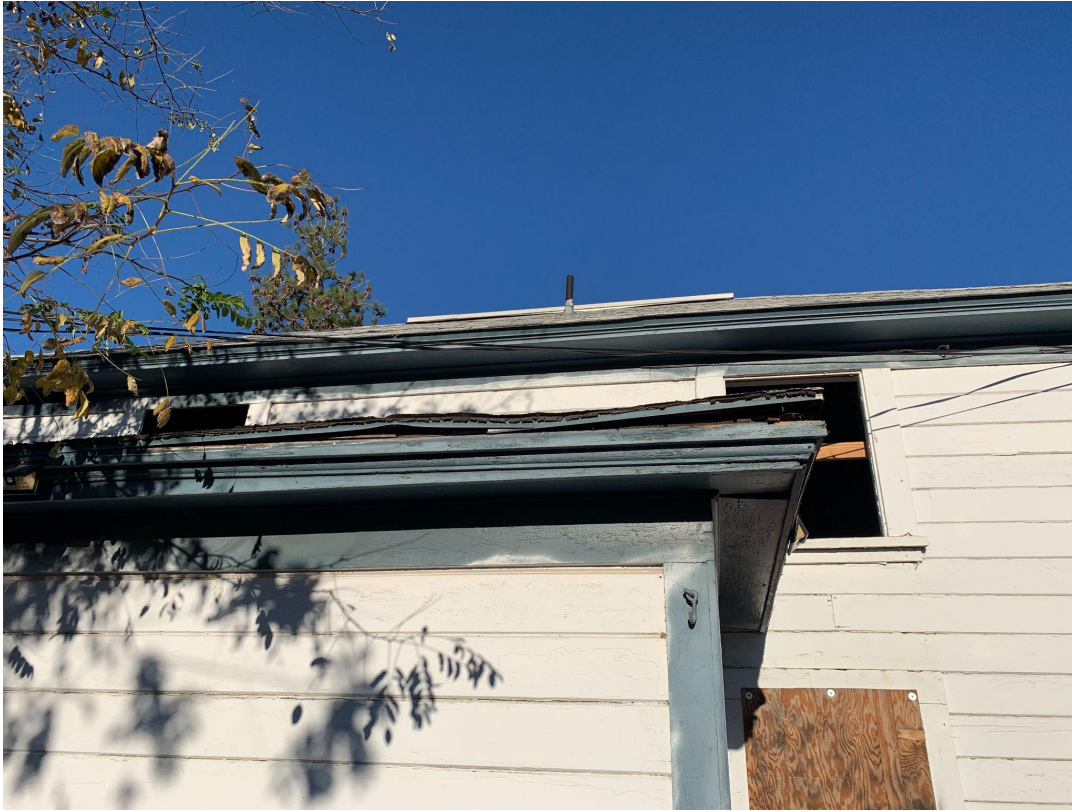
Figure 5. Entire roof has extensive dry rot, including the roof sheathing and roof rafters. High likelihood of collapse under any sort of load.
