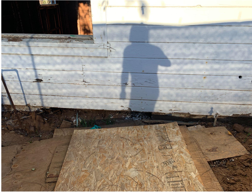
Figure 3. Exterior View (Existing wood on grade foundation has completely rotted away; this wall has no structural support.)
