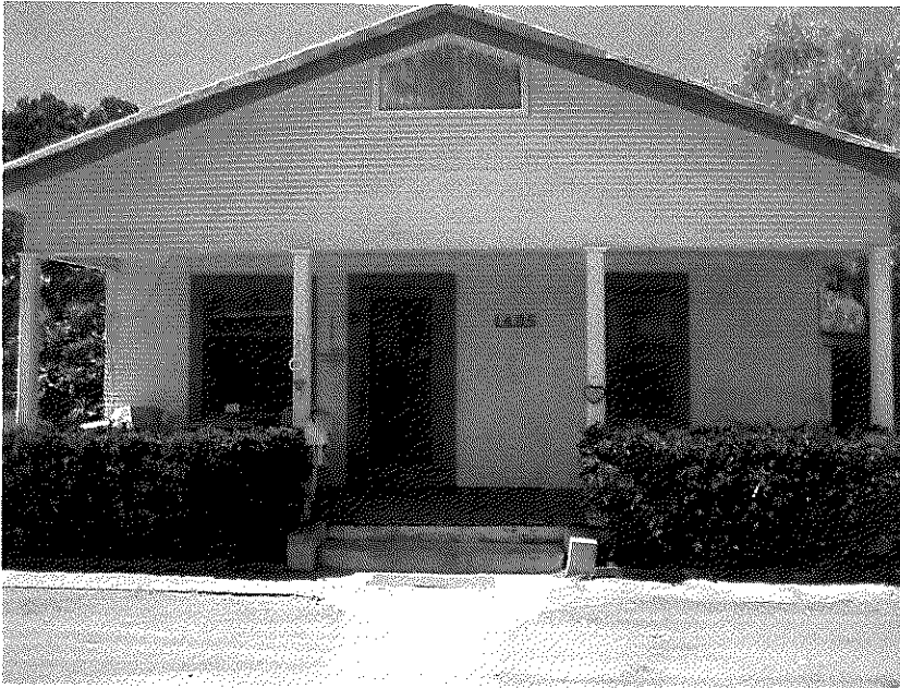
Photograph #3 East Elevation View Facing West
