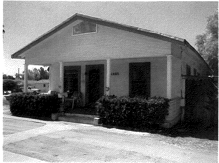
Photograph #4 East & North Elevations View Facing Southwest
