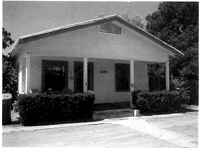
Photograph #2 East Elevation View Facing West
