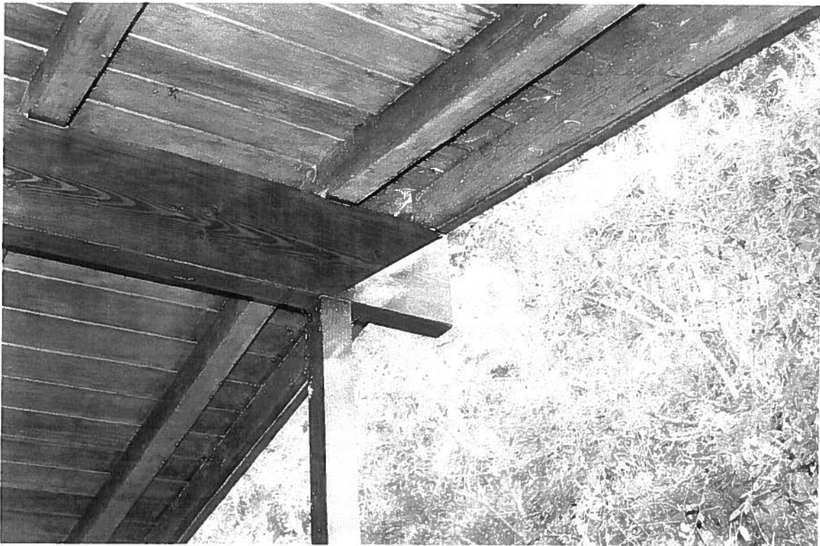
Massive beam supporting rear roof extending over porch
