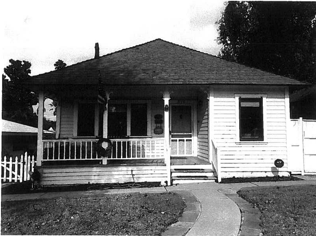
Front/south elevation showing front entry and porch
