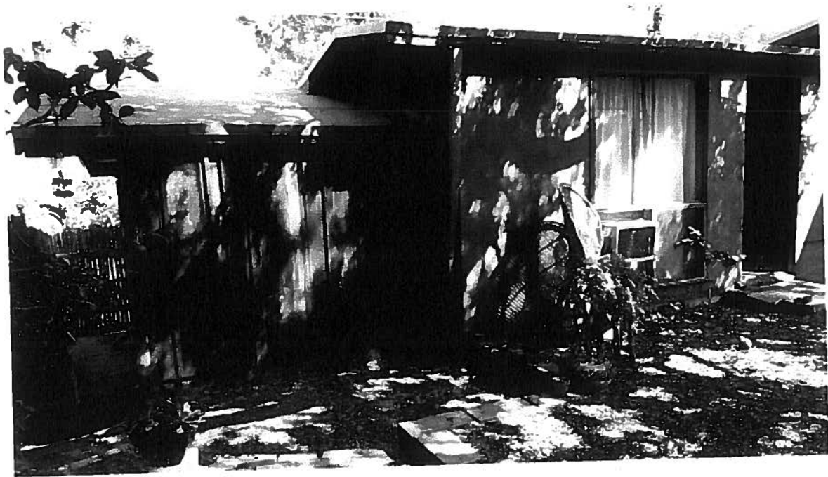
South wall of garage with access to bedroom, board and batten disguises shallow storage cabinets to the left.
