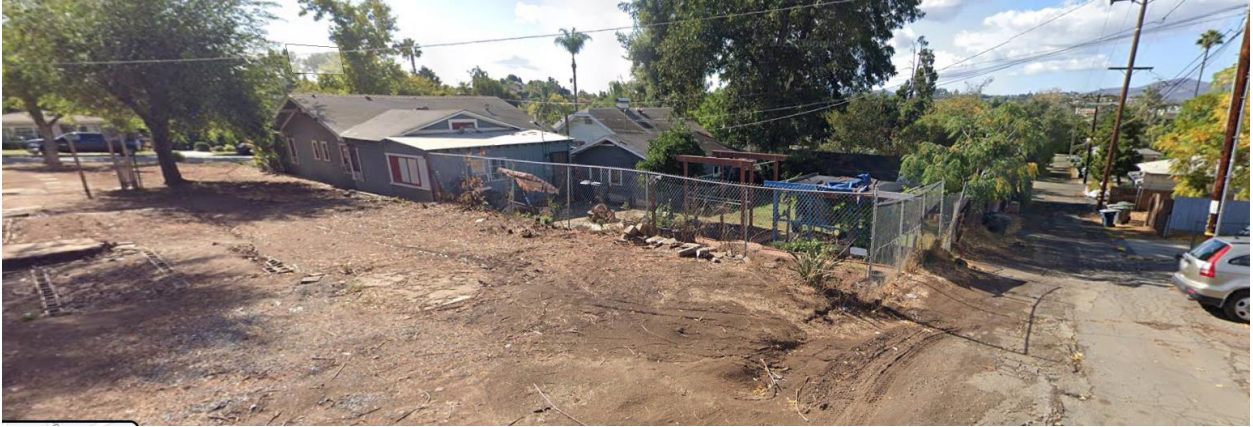
Pad area for proposed garage with east view of alley and adjacent house.
