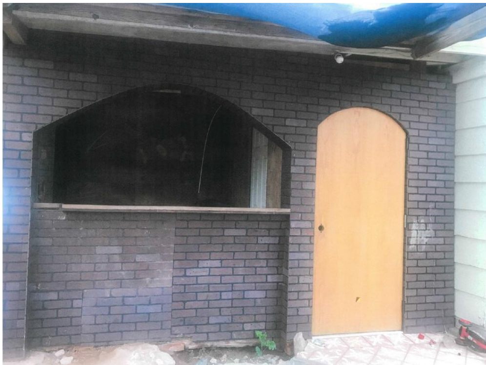
SOUTH SIDE VIEW OF ENCLOSED PATIO
