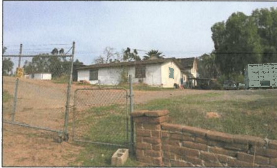
Original Upper Gate
