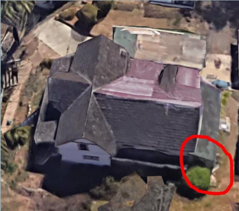
Past Google aerial view
