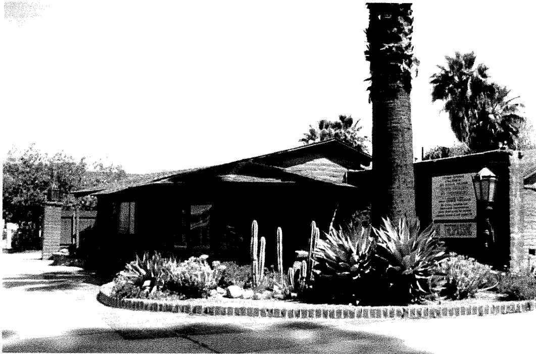
Image 5: Looking northeast. Note the period landscaping and six foot adobe site wall and scone.
