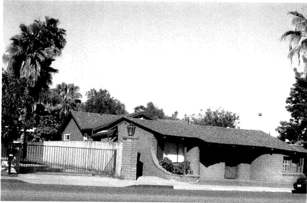
Image 3: Looking southeast at portions of north and west facades.
