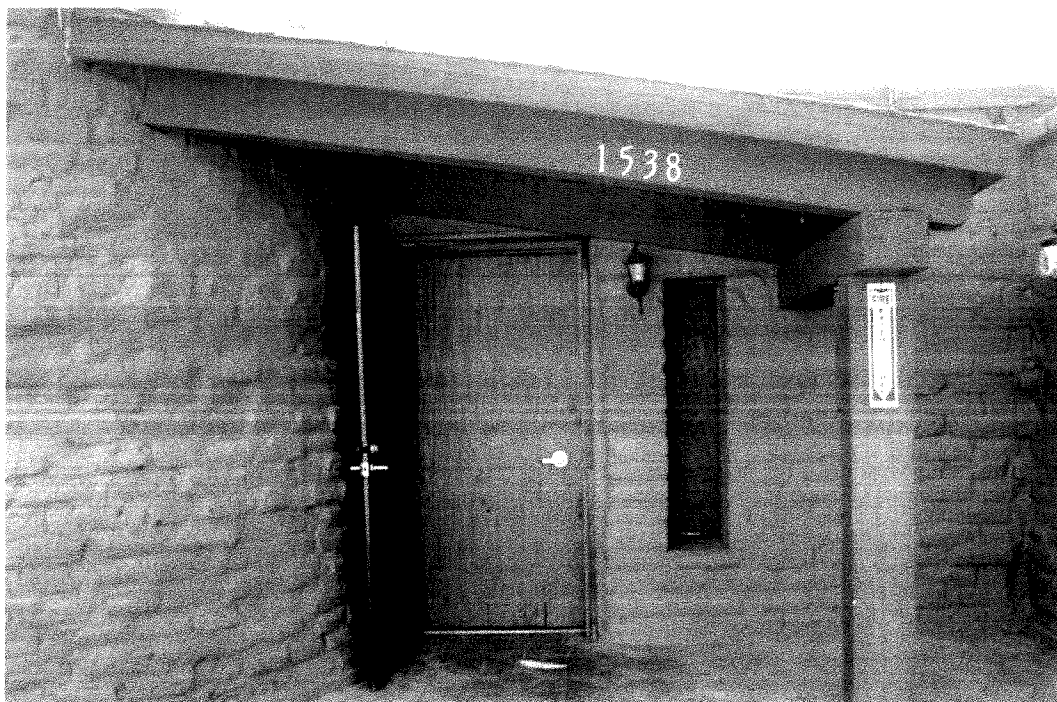
Image 10: Detail of the 1960 office entry with shed porch roof, heavy timbered square posts, and Mexican pavers. The original flush door is extant with recessed colored textured side lite.
