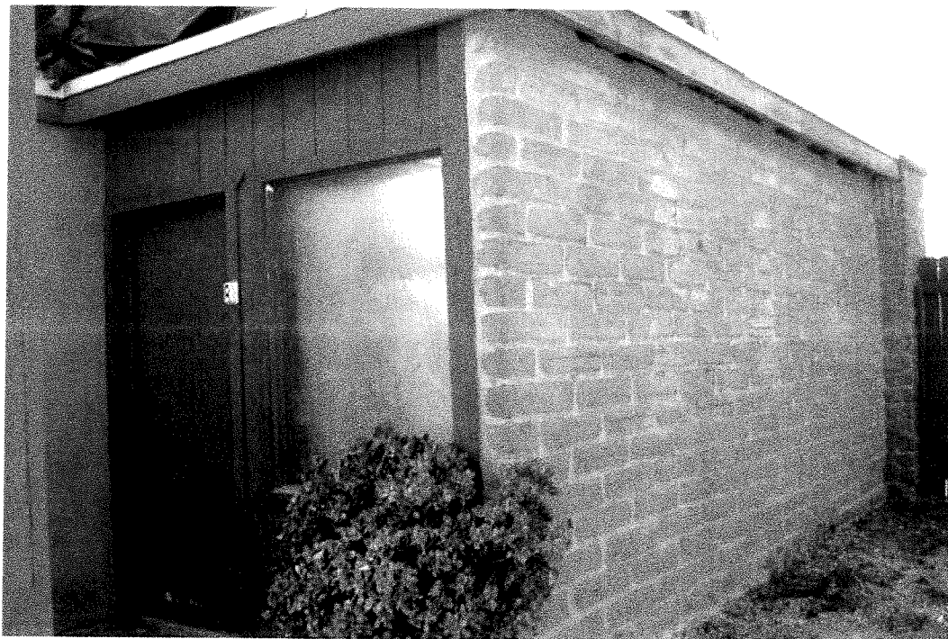
Image 12: Looking southeast at the 1957 adobe workshop (storage) building. The flush door and fixed window appear to be original.
