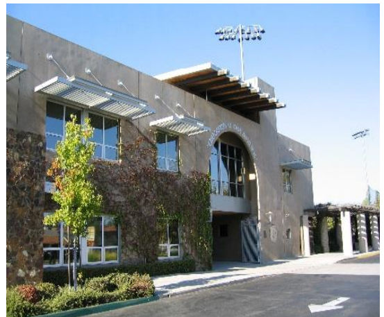
Source: City of Escondido
