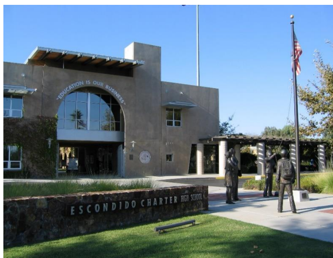
Source: City of Escondido
